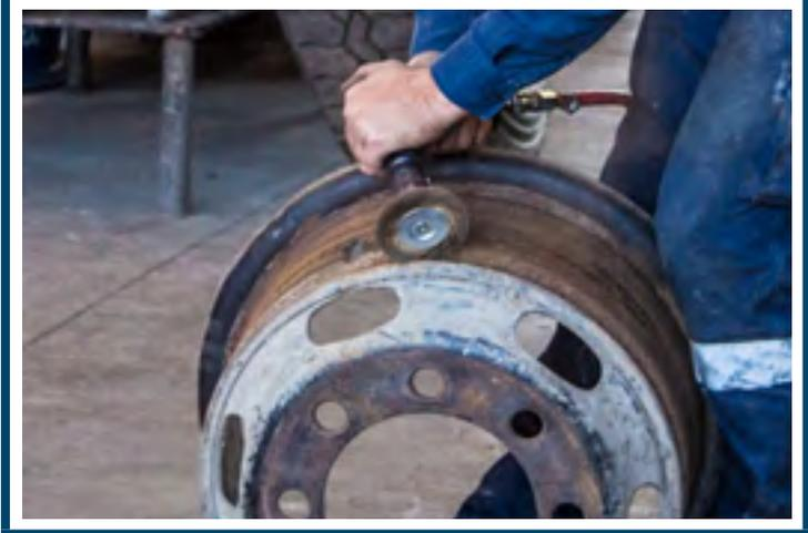
**Figure 11** Rejected rims are identified and isolated
