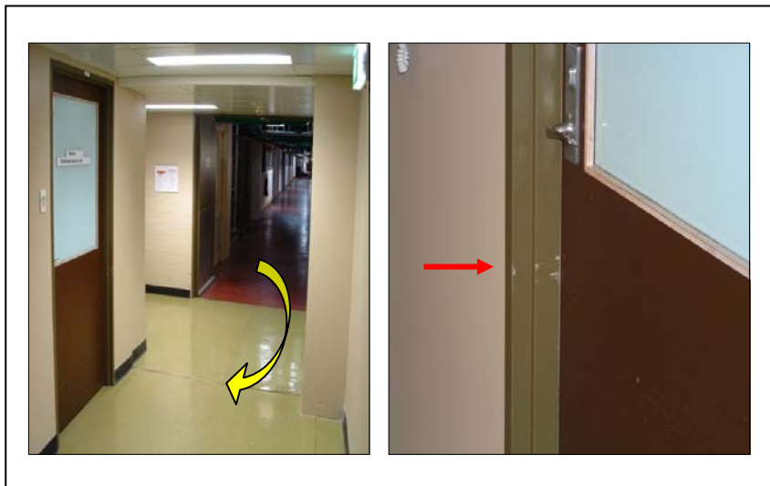
View of mortuary corridor where turning a bariatric bed or trolley carrying a bariatric patient in through the mortuary door is difficult
