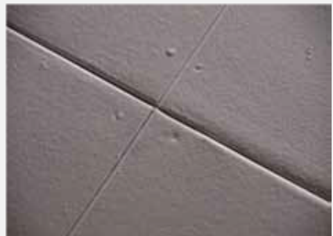
Figure 8 Examples where fasteners are fixed into the LDB sheeting and the edges are bevelled or slanted
