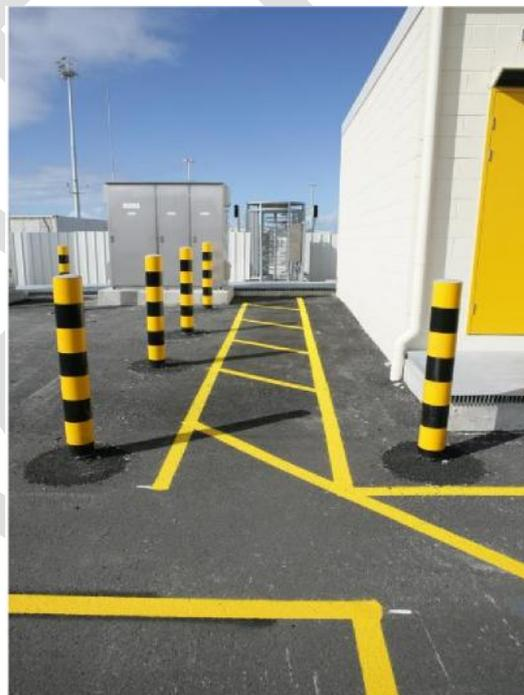
**Figure 1:** Walkway marked with lines and bollards
