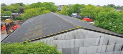
AC roof and wall cladding (non-friable)
