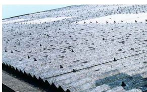
Non-friable - Contained in roof sheeting
