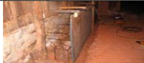
Asbestos cement (AC)
